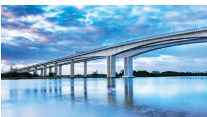
Monitor infrastructural deterioration in bridges
